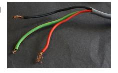
If you notice a green, gooey substance leaking from your sockets or switches, it could be a sign that you have this type of wiring. This "green goo" is an irritant, so avoid touching it. Have your wiring tested, as in some cases, a full rewire might be necessary.
